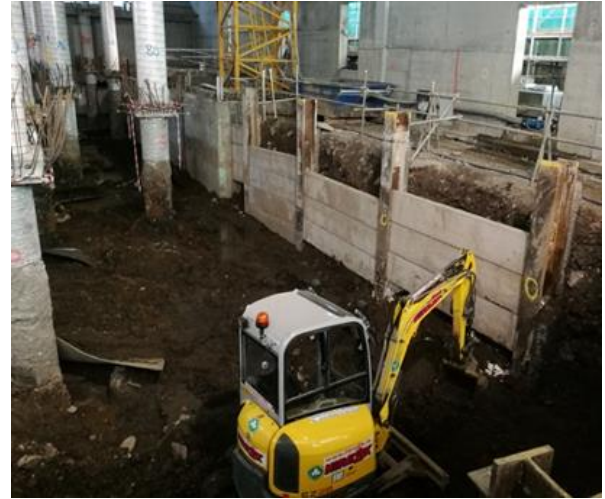
Figure 7. Kingpost wall installation.
